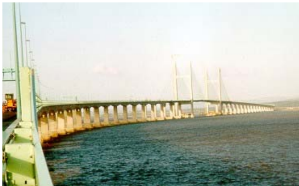
Second Severn Crossing
